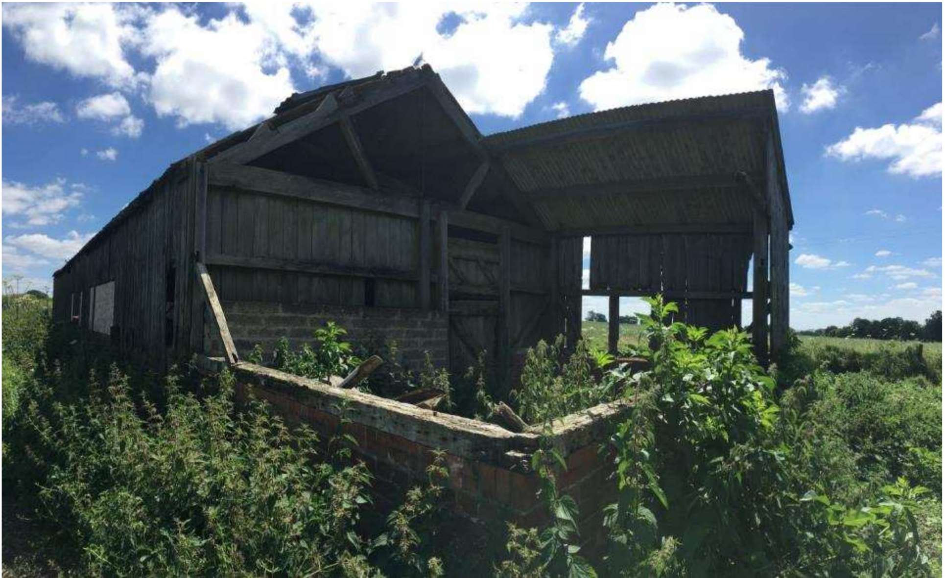
View of South (side) elevation of Barn No. 1
