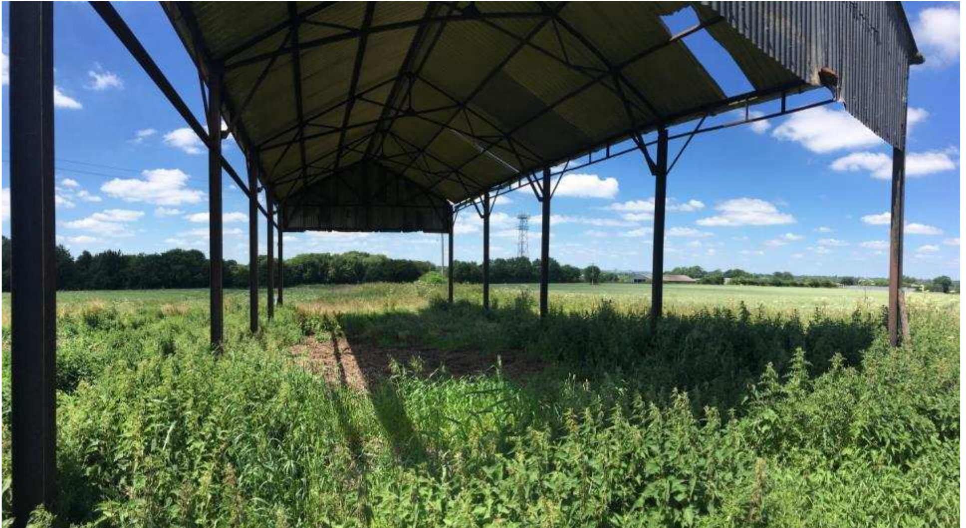
View inside Barn No. 2
